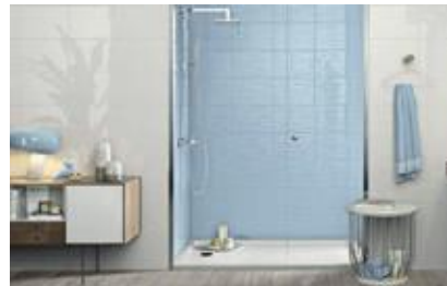
In the main bathroom: acrylic shower tray made by ROCA and glass shower screen with a fixed panel.
